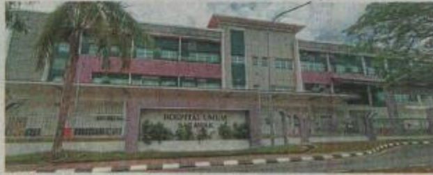
Ready to go: The Sarawak General Hospital has been working hard to build the hospital's capacity of its Phase I-equipped Clinical Research Centre. — Others
